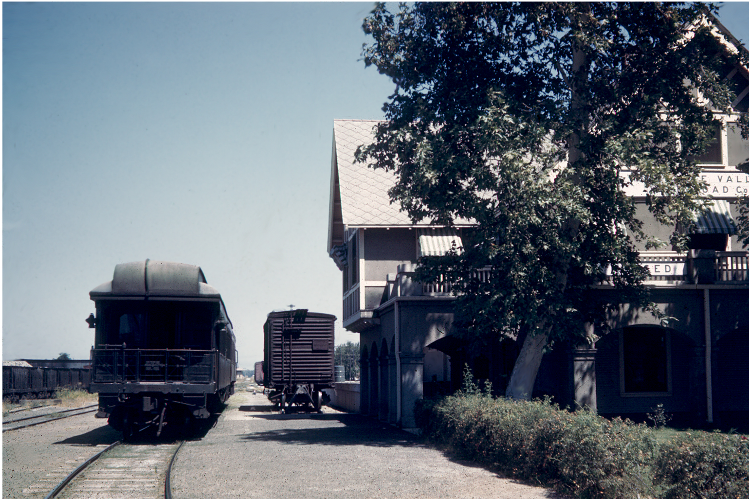
Another view of the station at the time of the September 1944 fan trip.
